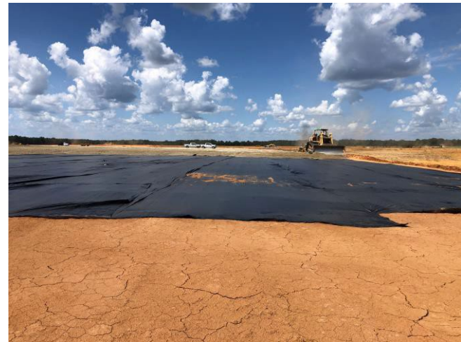
July 29, 2022: Fabric and Stone Placement for the South Laydown Yard
