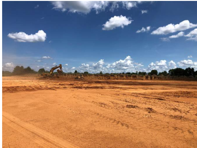
July 28, 2022: Excavation Ongoing in the Borrow Pit
