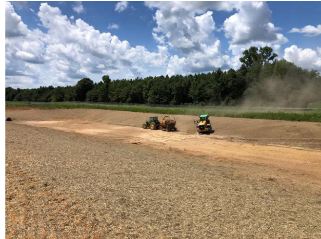
July 28, 2022: Seeding and Mulching Ongoing in the Detention Pond
