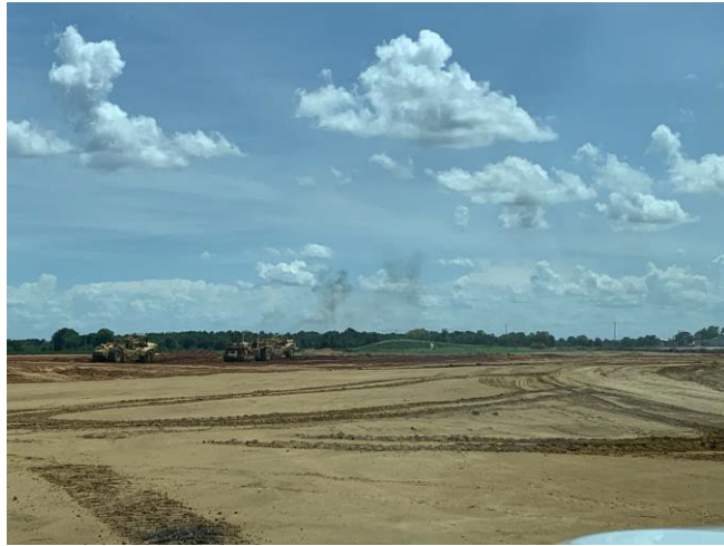
July 26, 2022: Grading Ongoing in Quadrant C206
